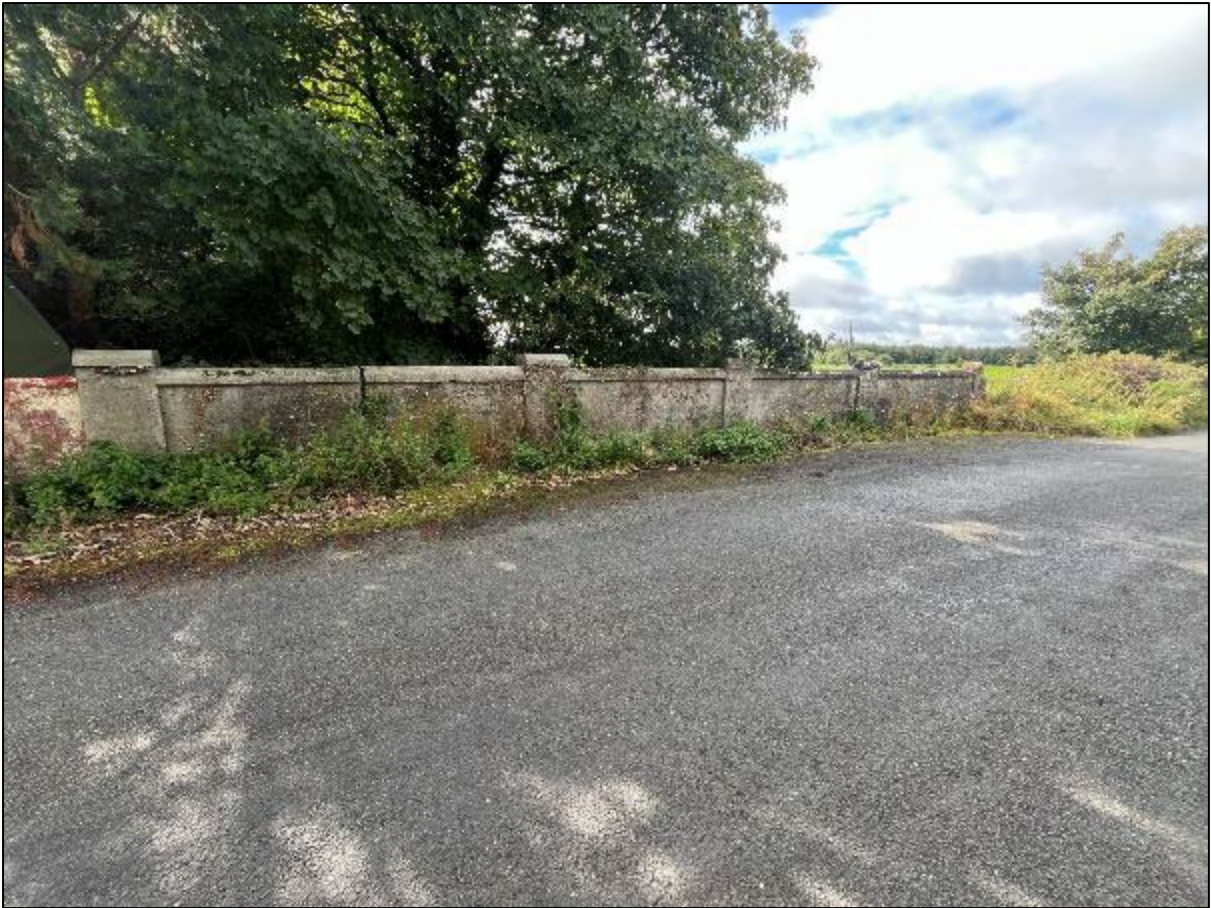
Plate 14.12: View of Bridge TN042-027---- on grid connection route
